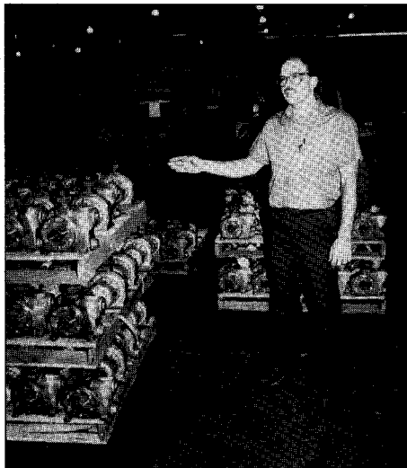
Figure 2. Dewey Gross, a workshop presenter and plant tour guide, discussed pumping unit cell operations.
